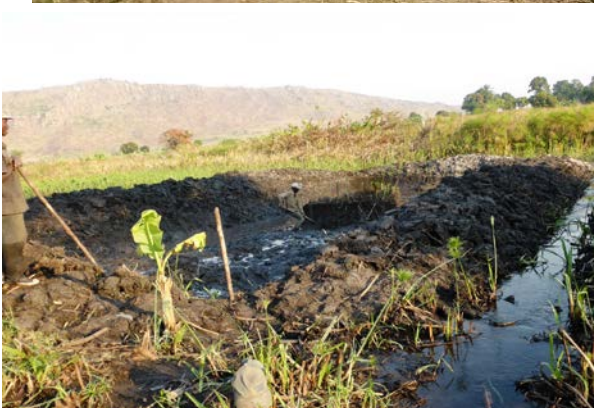
Earthen fish ponds in construction
