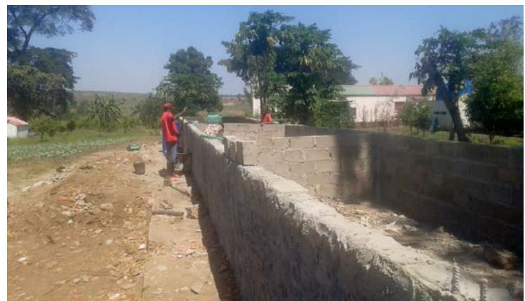
After (concrete fish pond in construction)
