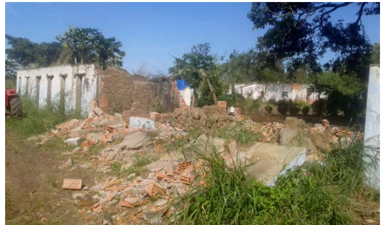
Before (demolition of the old structure)
